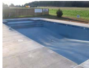
Pool Before Water was added
